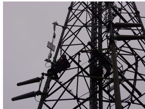
Figure 2: An engineer panning a flat plate antenna
